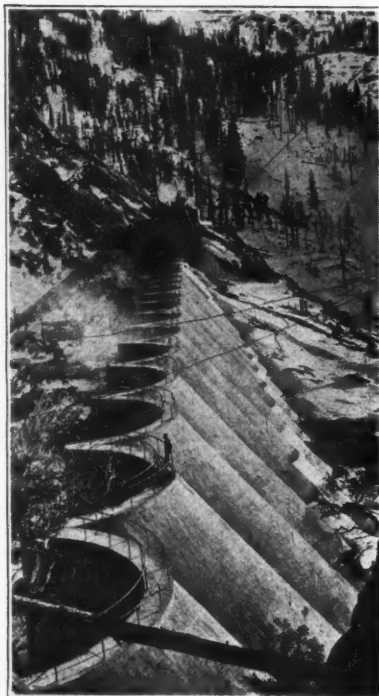
Top of Dam
